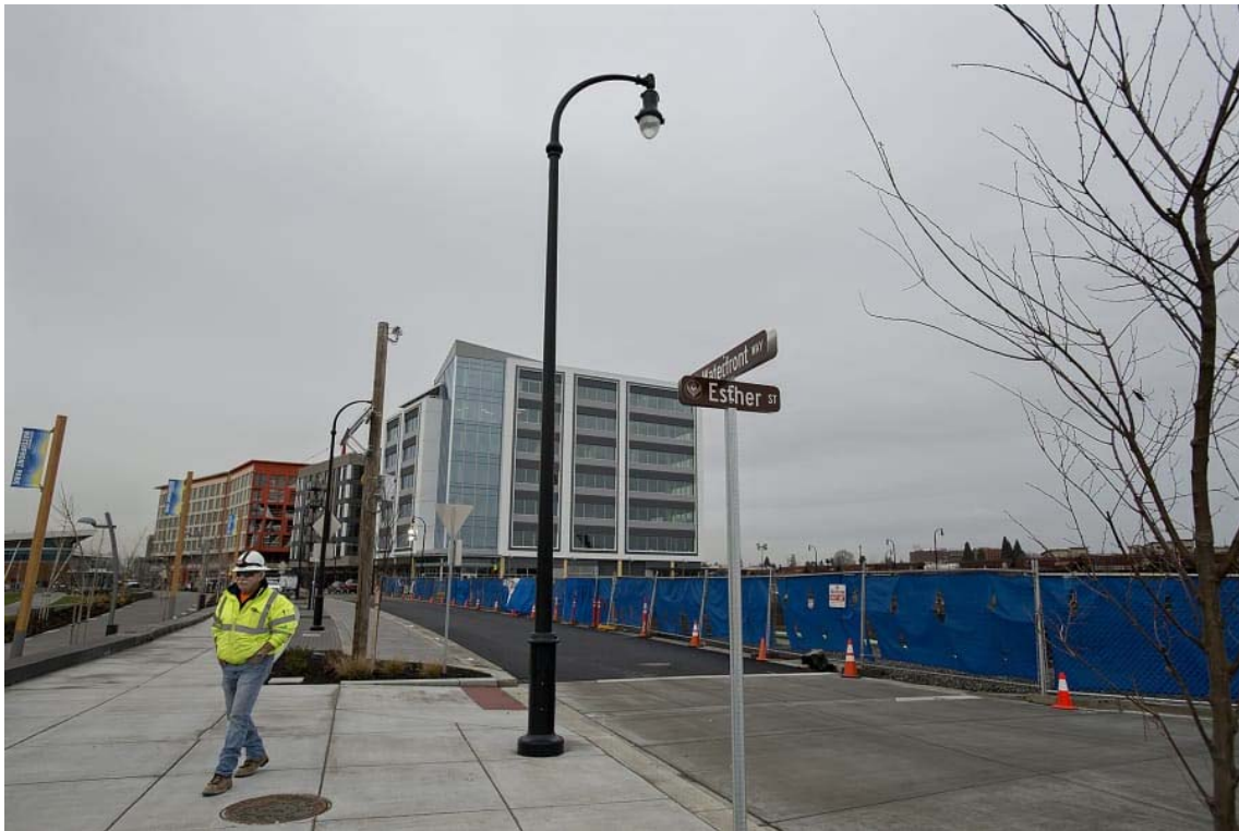
Project superintendent James Fuller of Kirkland Construction Group walks past the future site of the Kirkland Tower and Hotel Indigo. A crane necessary to the buildings' construction is being assembled at the site. Amanda Cowan/The Columbian
